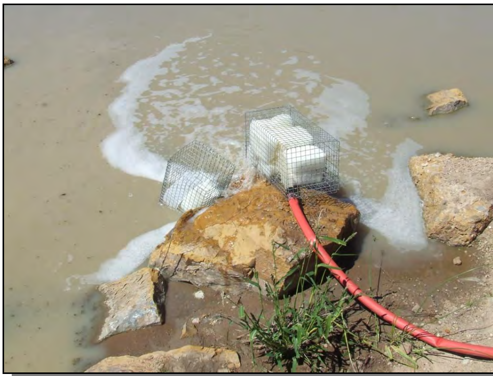
Plate 2 - Flocculant Blocks Used in SD3
